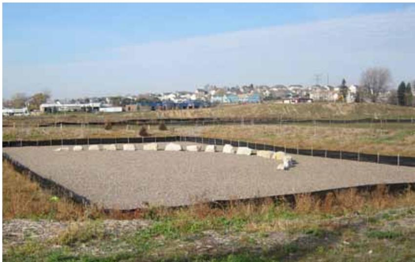
SAND FILTER ENHANCED WITH IRON FILINGS TO REMOVE DISSOLVED PHOSPHORUS FROM STORMWATER (MAPLEWOOD, MN).
